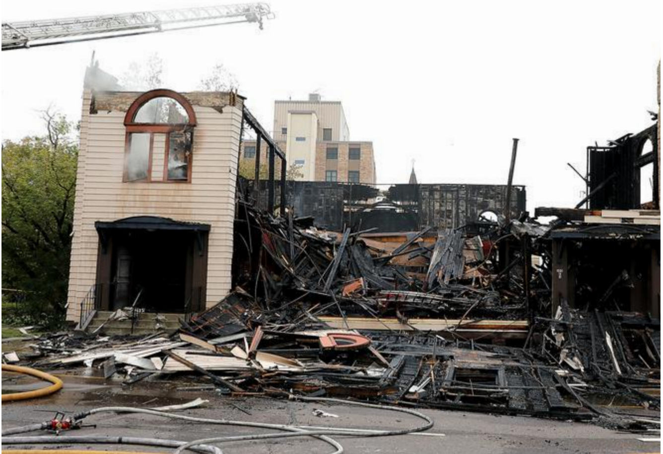
Smoke still rolls out of a window after fire destroyed the Adas Israel Congregation synagogue Monday in Duluth. Jed Carlson / Forum News Service
